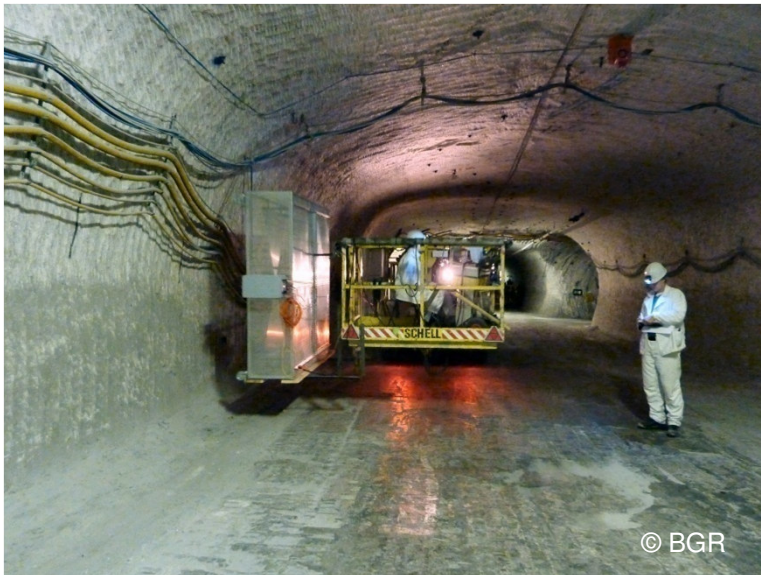
GPR measurements in the wall of a drift at the 840-m level
