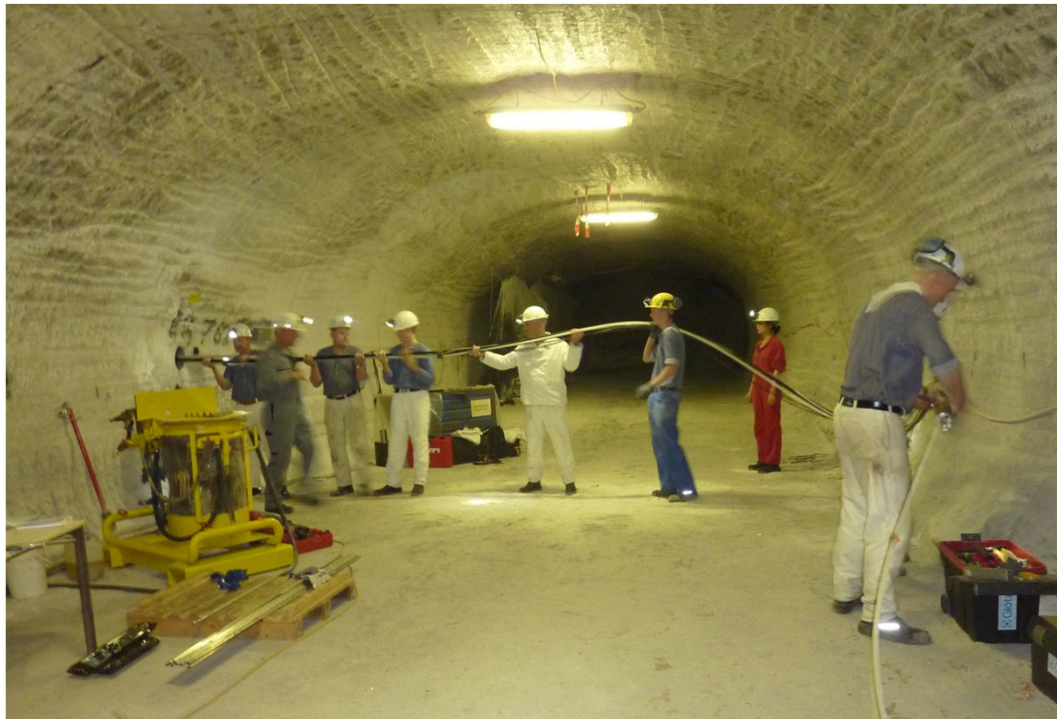
Installation of an extensometer at the 840-m level
