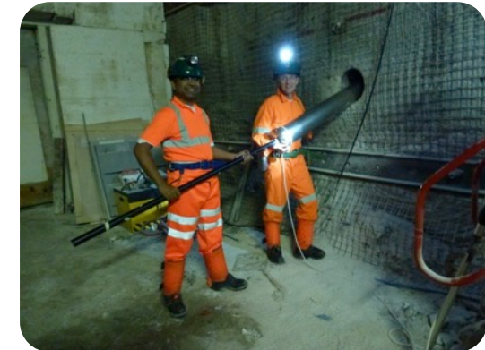
Bore hole detector installation
