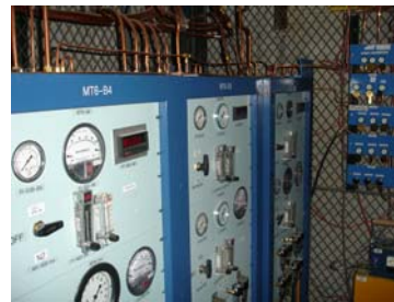
Gas delivery to 6 locations
