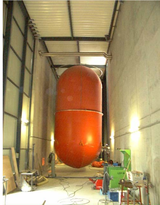
installation of gas bags
