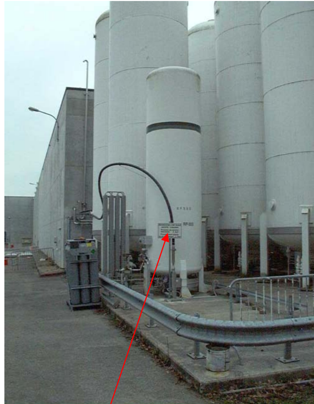
Removal of 6000 l LN2 reservoir behind SUH8 and reconnection cryoplant
