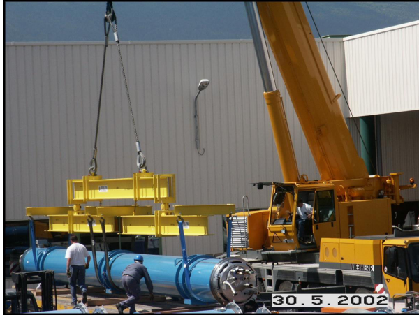
Figure 3: Liebherr Mobil crane 160 t
