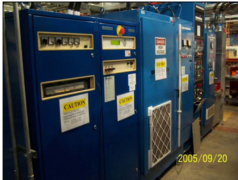
Ring RF equipment in Ring service building
