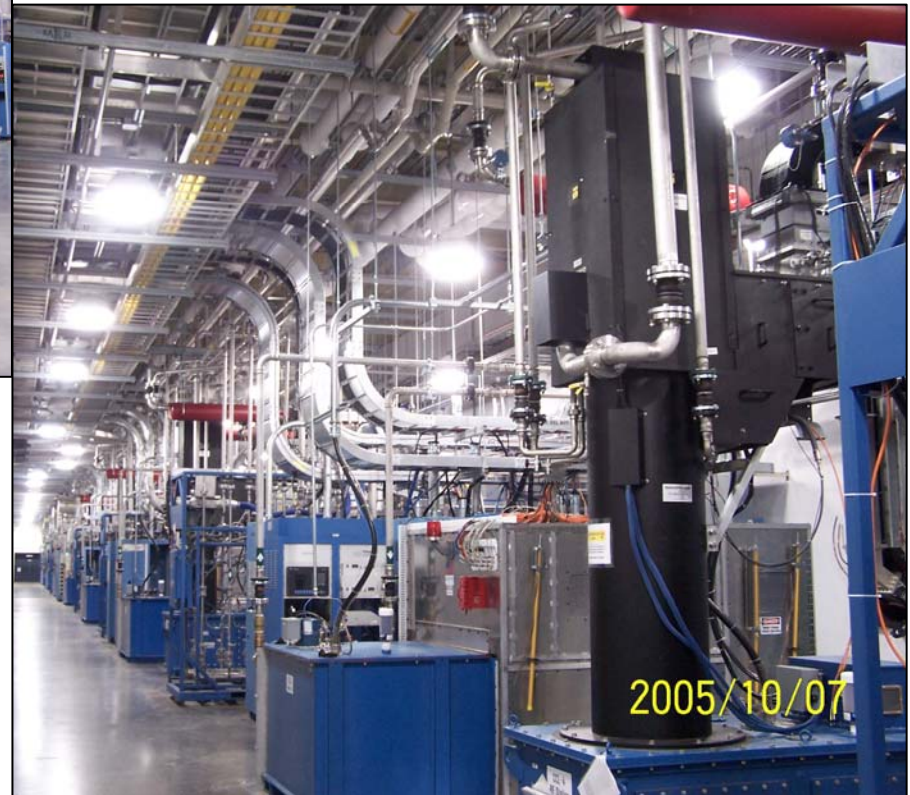
Four 805 MHz, 5 MW klystrons power the CCL
