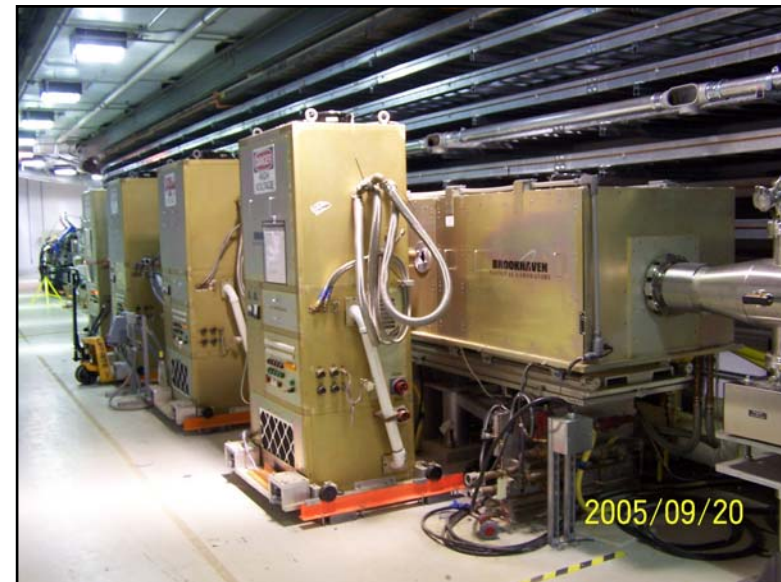
Ring RF cavities and amplifiers in Ring tunnel
