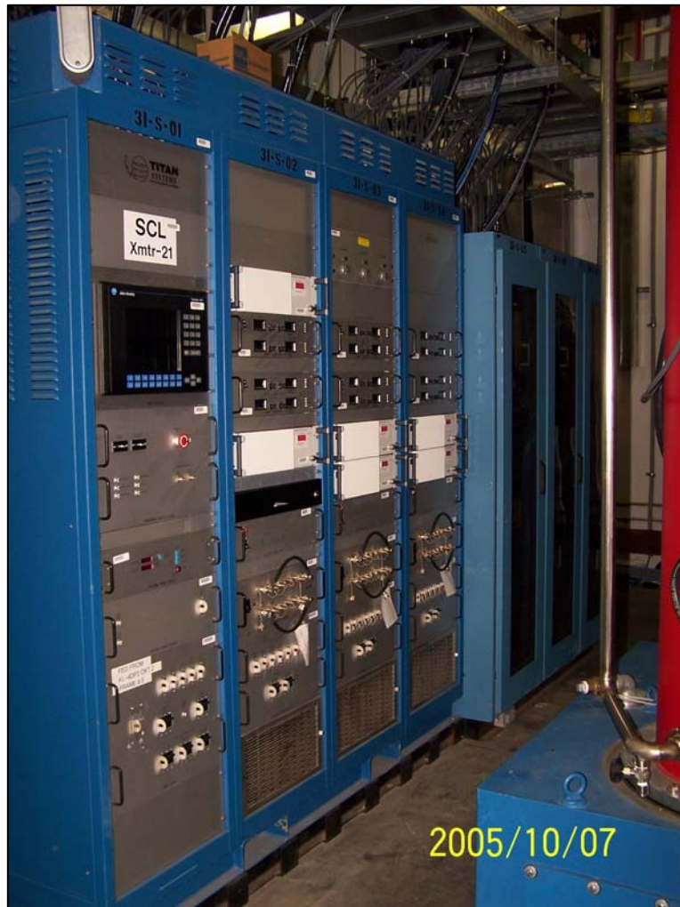
Transmitter racks & LLRF for support of six klystrons.
