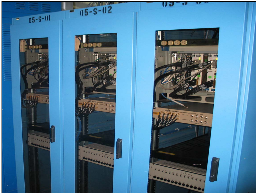
Typical LLRF control rack installation in the superconducting linac.
