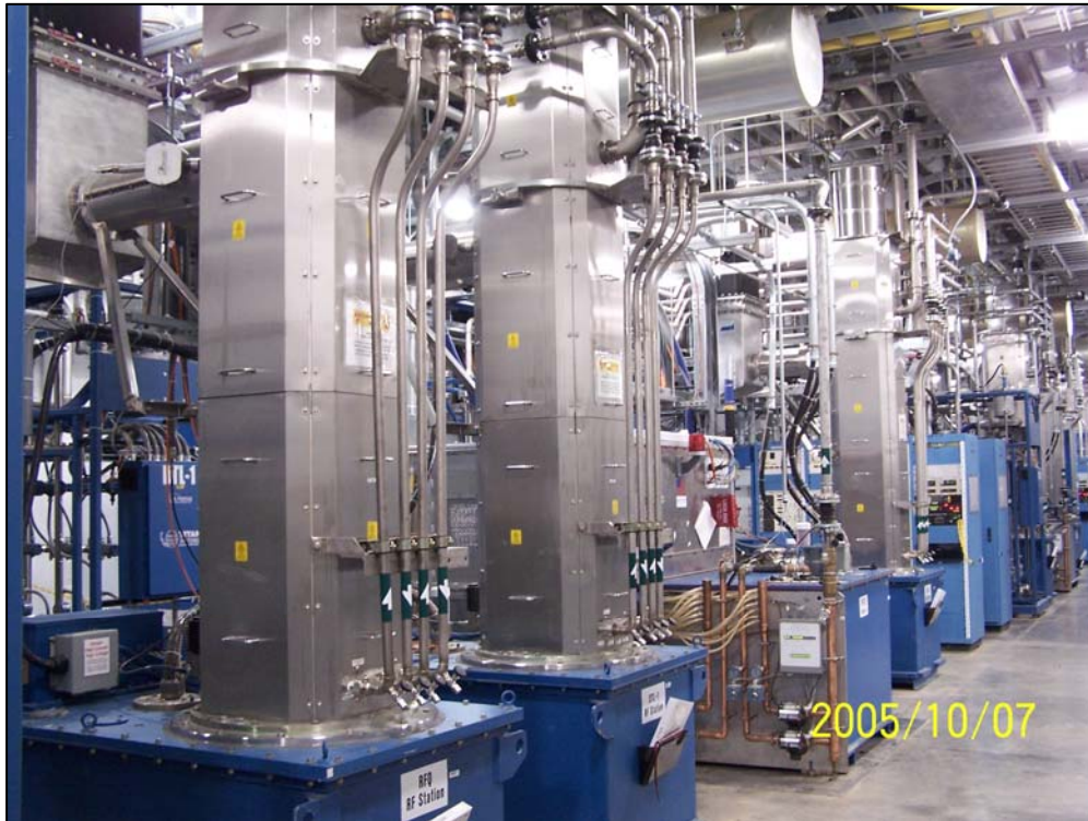
Seven 402.5 MHz, 2.5 MW klystrons power the RFQ and DTL
