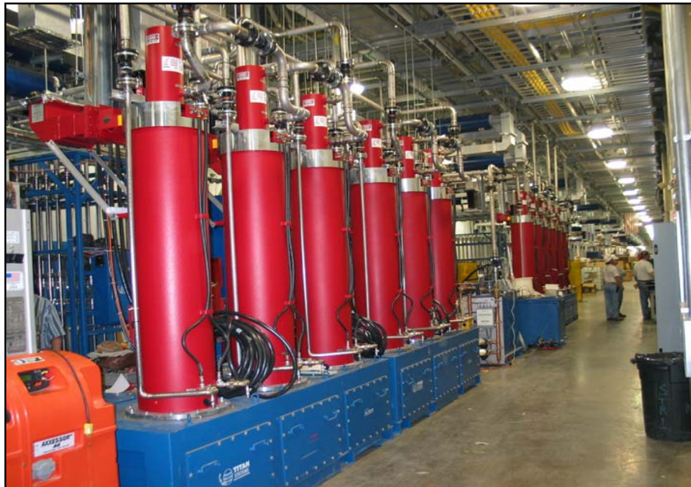
Linac klystron gallery during installation of baseline RF systems
