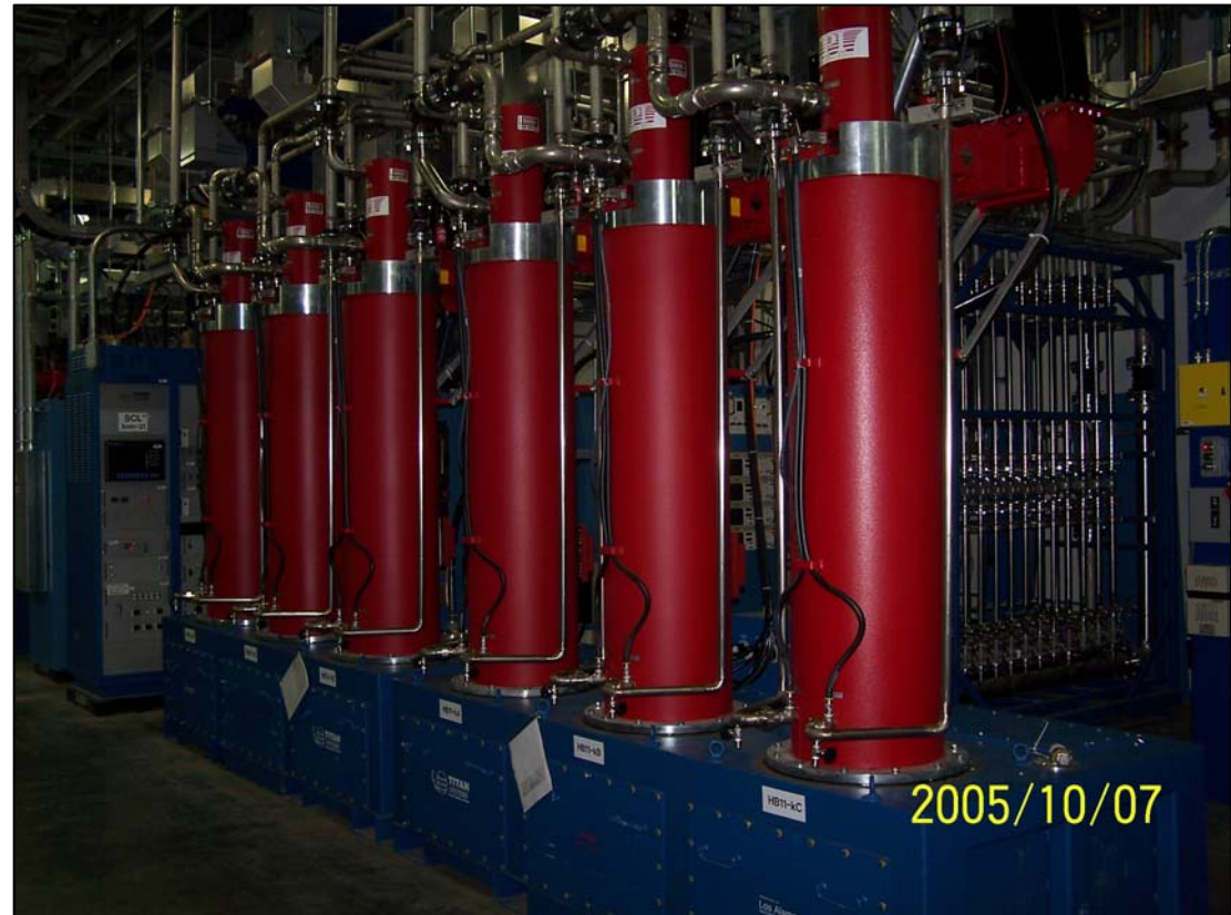
Three klystrons mount to a single oil tank.
