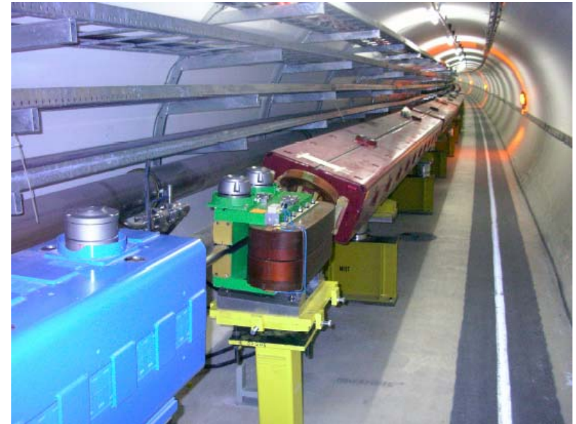
TI8 completed and partly tested
