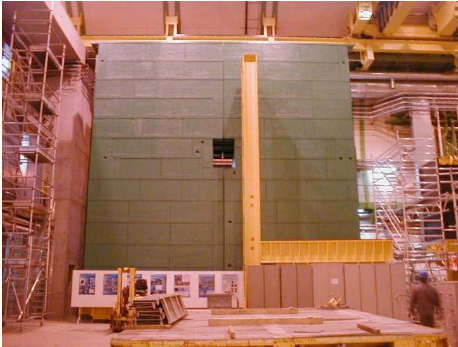
First three Muon filter wall assembled
