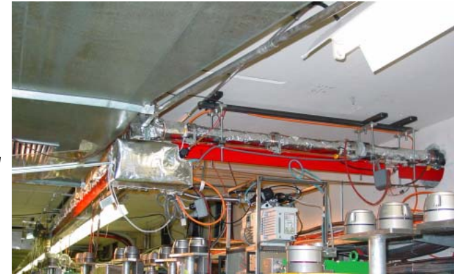
17m waveguide with 5 bends but low-loss (85% transmission) (Russian collaboration)
