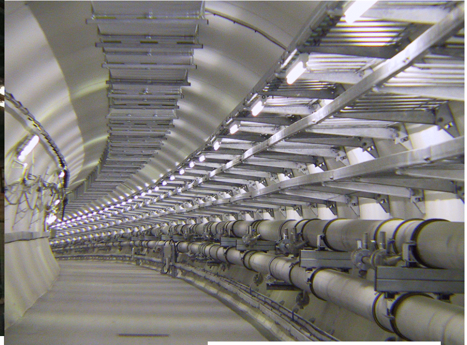
Proton beam tunnel Feb. 2005
