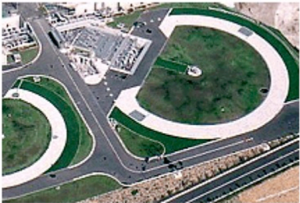
Bird's-eye view of underground storage tanks
