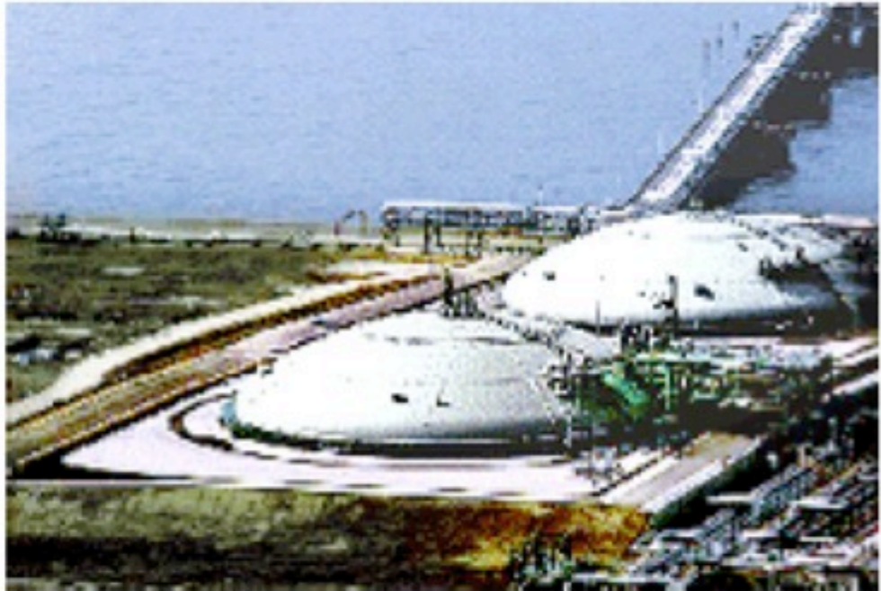
Bird's-eye view of in-ground storage tanks
