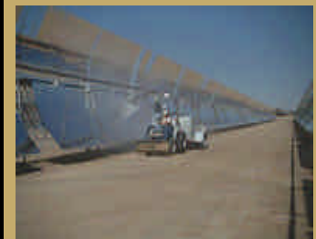
O+M Solar Field
