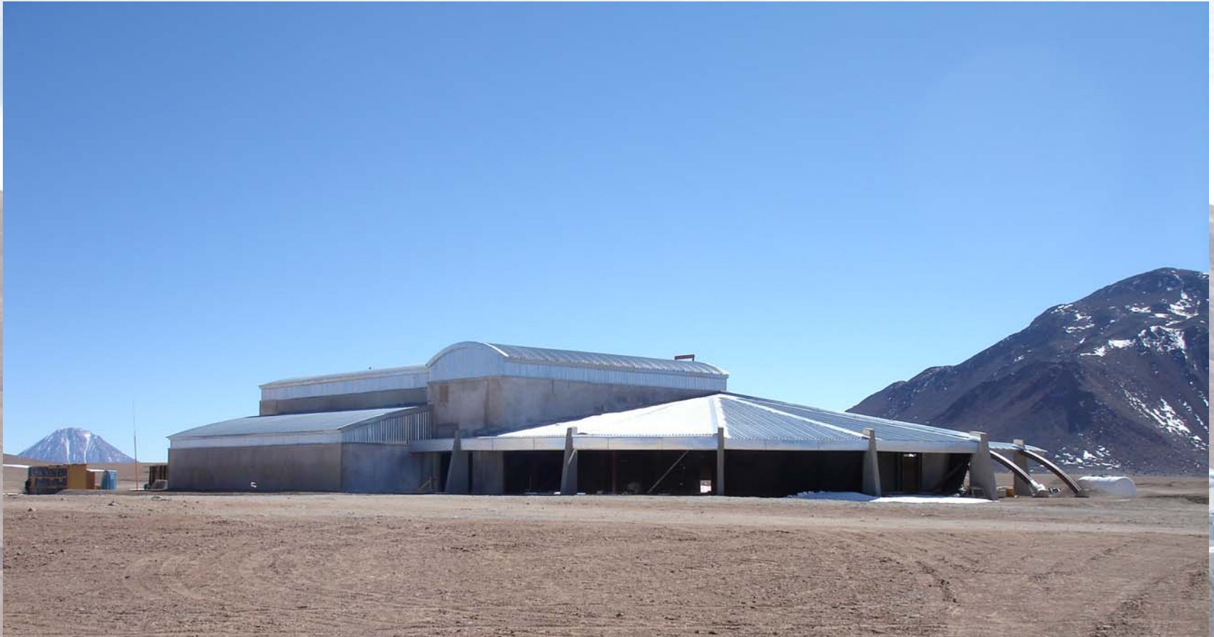
The AOS Technical Building– July 2006
