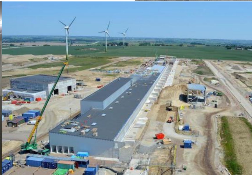
Linac tunnel completed
