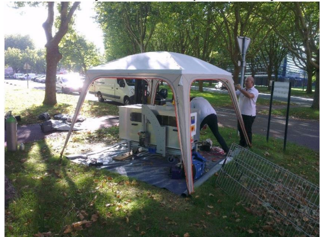
Battery and solar panel only
