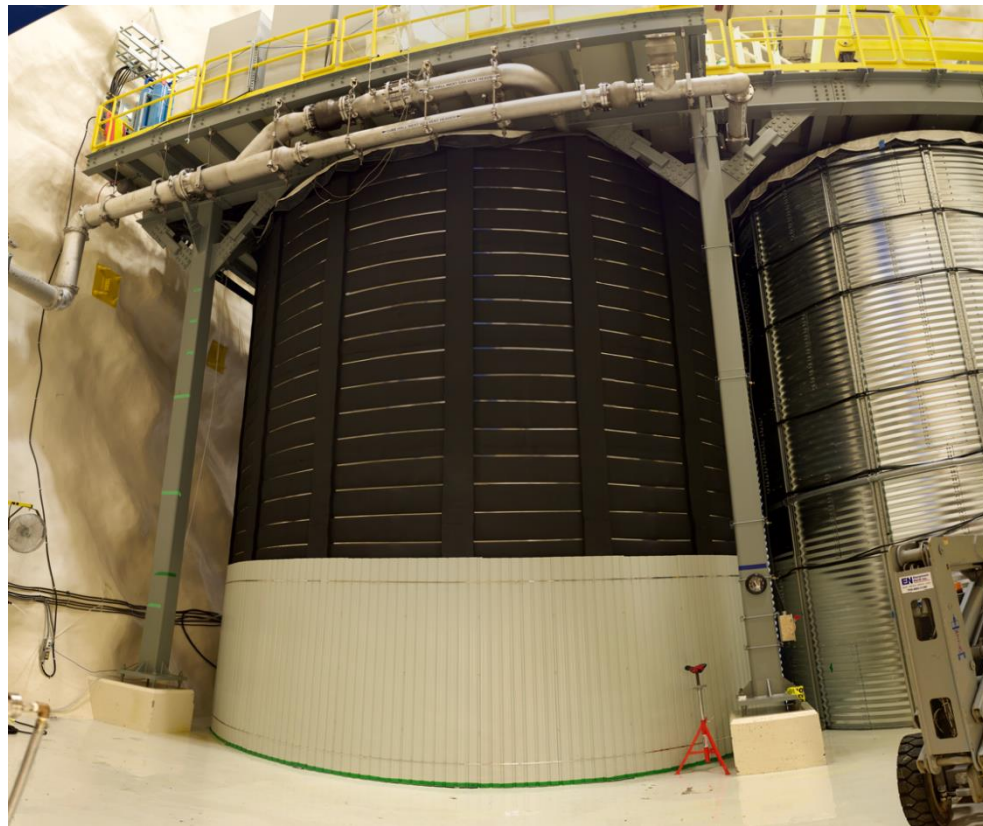
Shield Tank and emergency vent lines, tank was filled with water Oct 2015, cooldown started Feb 2016
