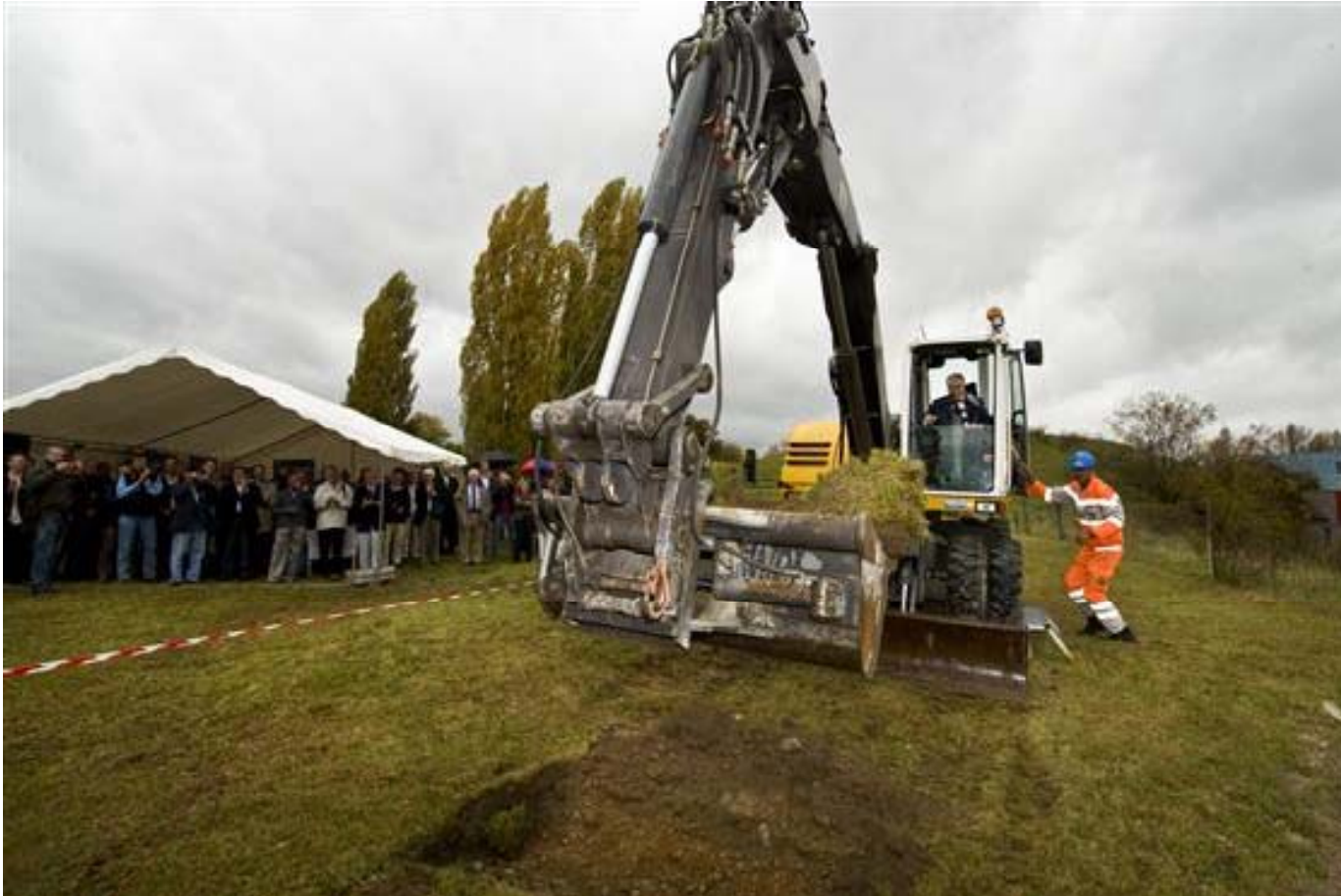
16 October 2008, Linac4 Groundbreaking by CERN Director, R. Aymar
