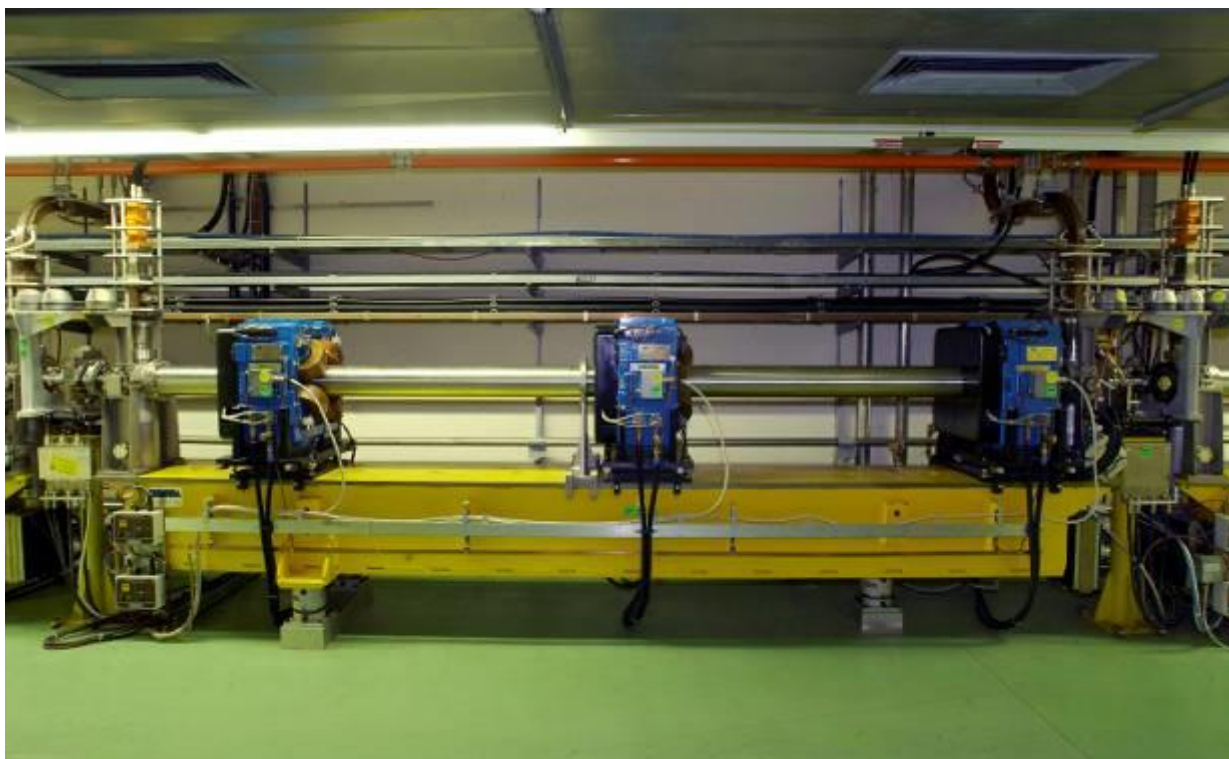
A 3 GHz LIL accelerating structure used for CTF3. It is 4.5 meters long and provides an energy gain of 45 MeV. One can see 3 quadrupoles around the RF structure.
