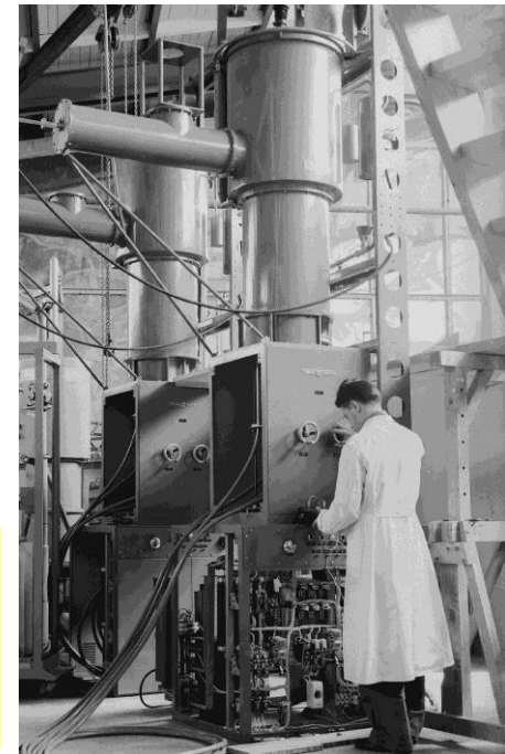
The CERN Linac1 triode amplifiers (2 MW, 202 MHz) in a photo of 1959
