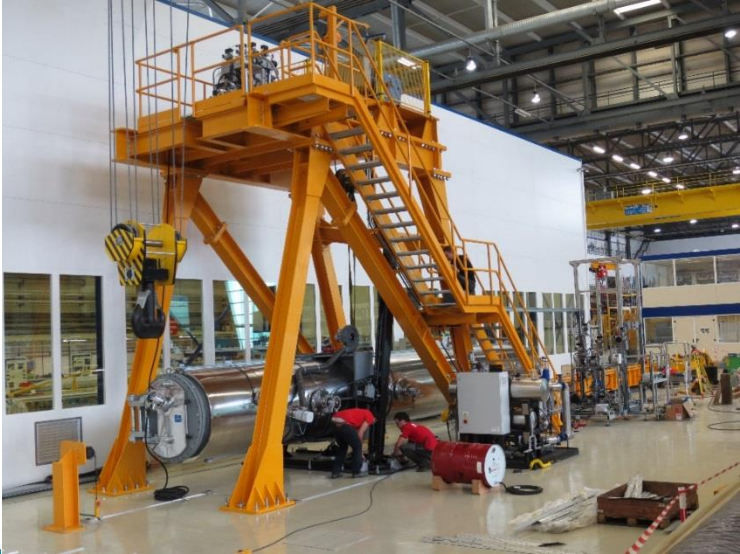
10.5 m long impregnation chamber
