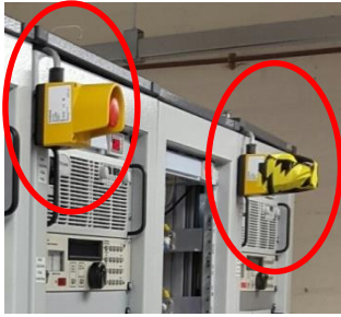
Emergency Off buttons installed on SS racks
