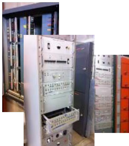
Legacy magnet interlocks for PS mains and auxiliaries
