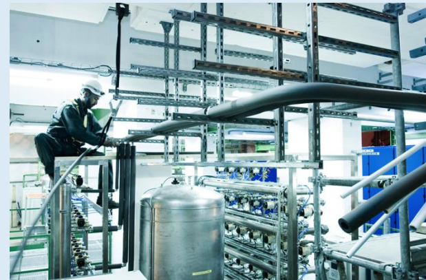
Cooling pipes to detectors installed by ALICE
