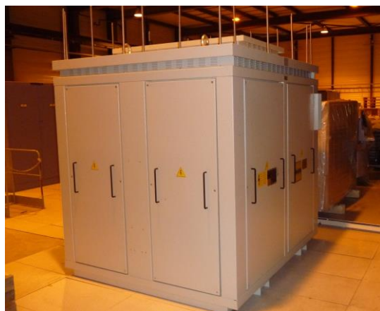
Cast Resin Transformer Type
