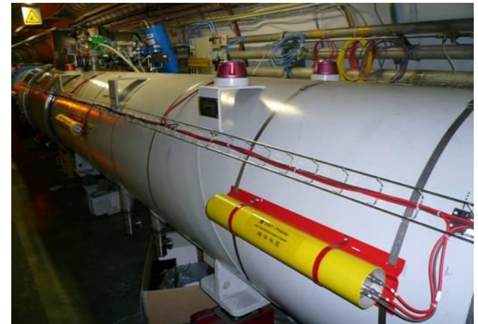
Beam Loss Monitor (BLM) in the LHC
