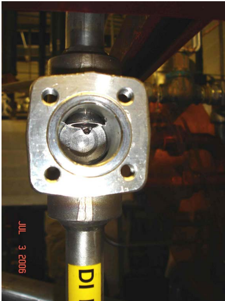
The gravity un-assisted check valve
