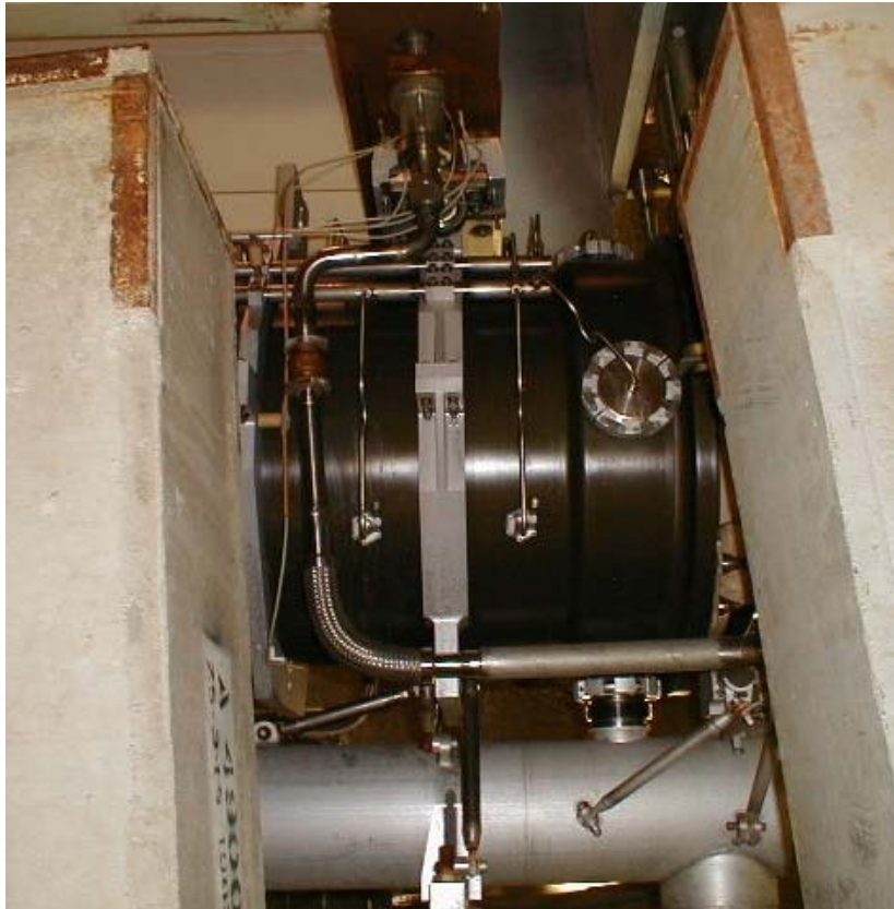
Set up temporary shielding with slot
