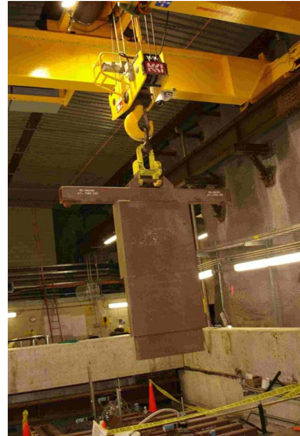
Steel shielding block being moved.
