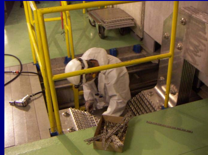
(with shielding in place)
