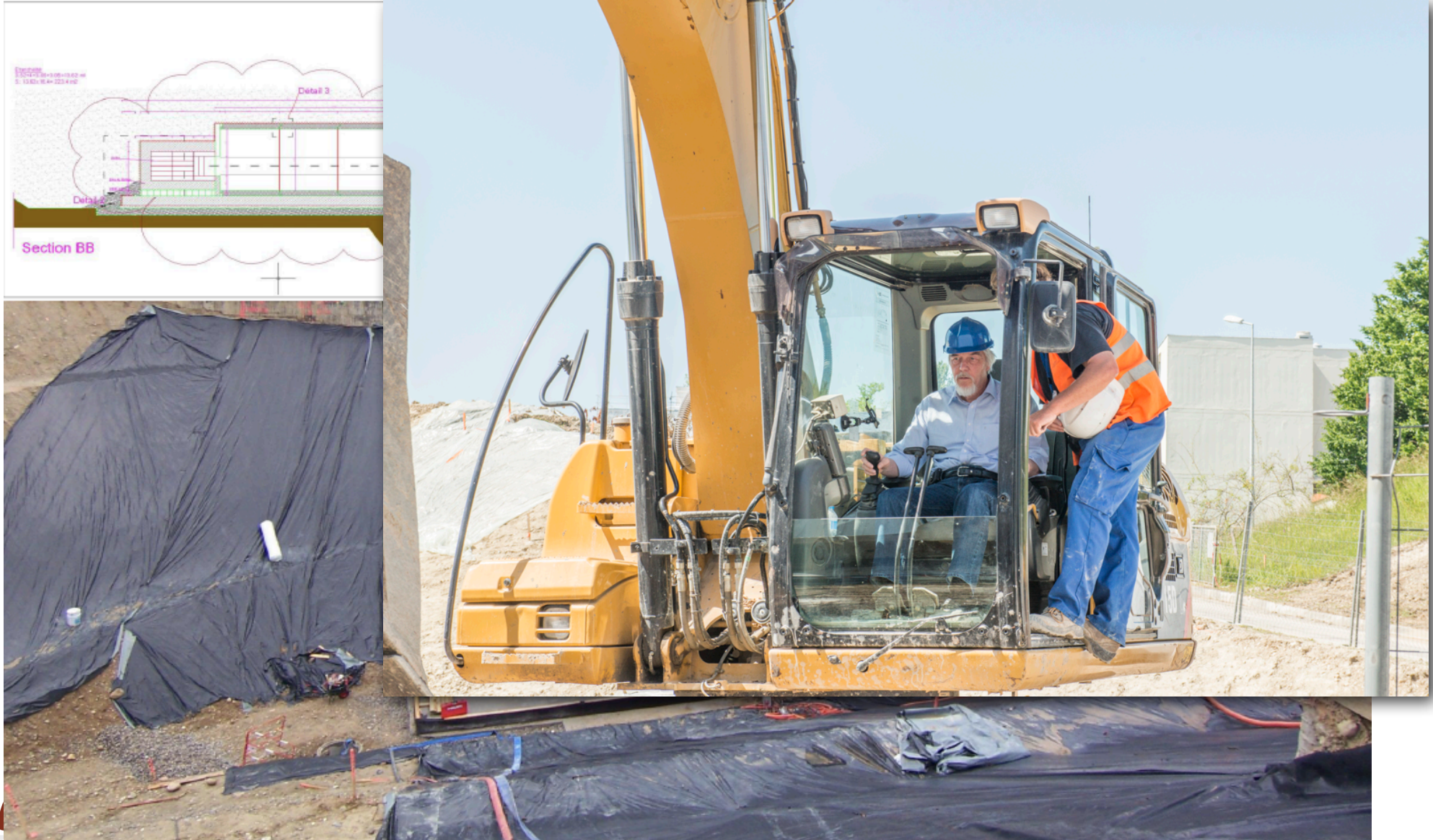
Excavation work for the new Beam Dump.
