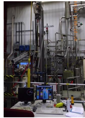
Vertical Magnet Test Facility
