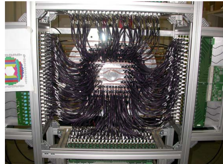
Electronics and cooling
