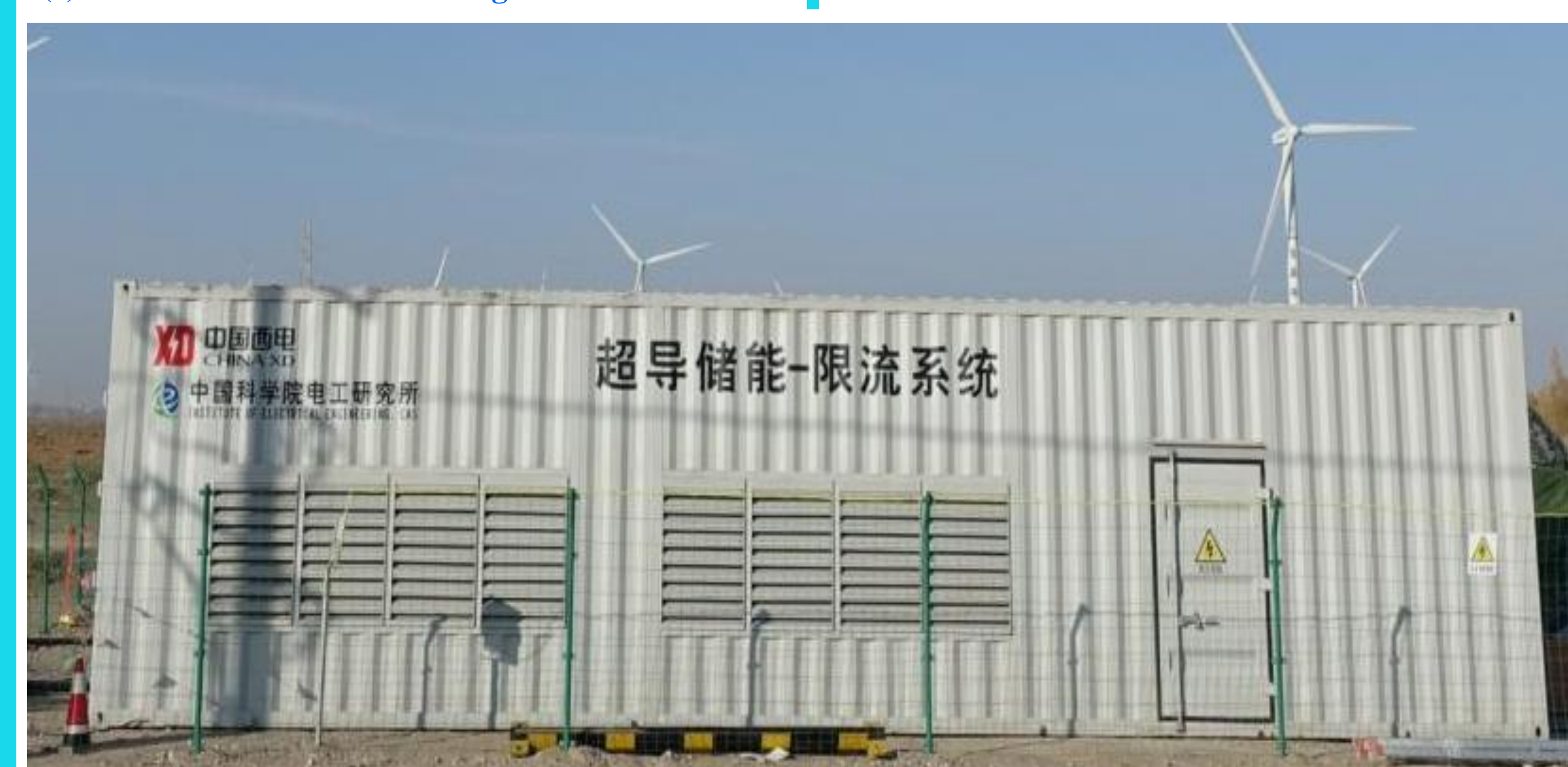
Fig.7. A photo of 1 MJ/1 MVA SMES-FCL installed and put into operation since January 6 of 2017 at a 10.5 kV wind farm locating in Yumen, Gansu Province of China.
