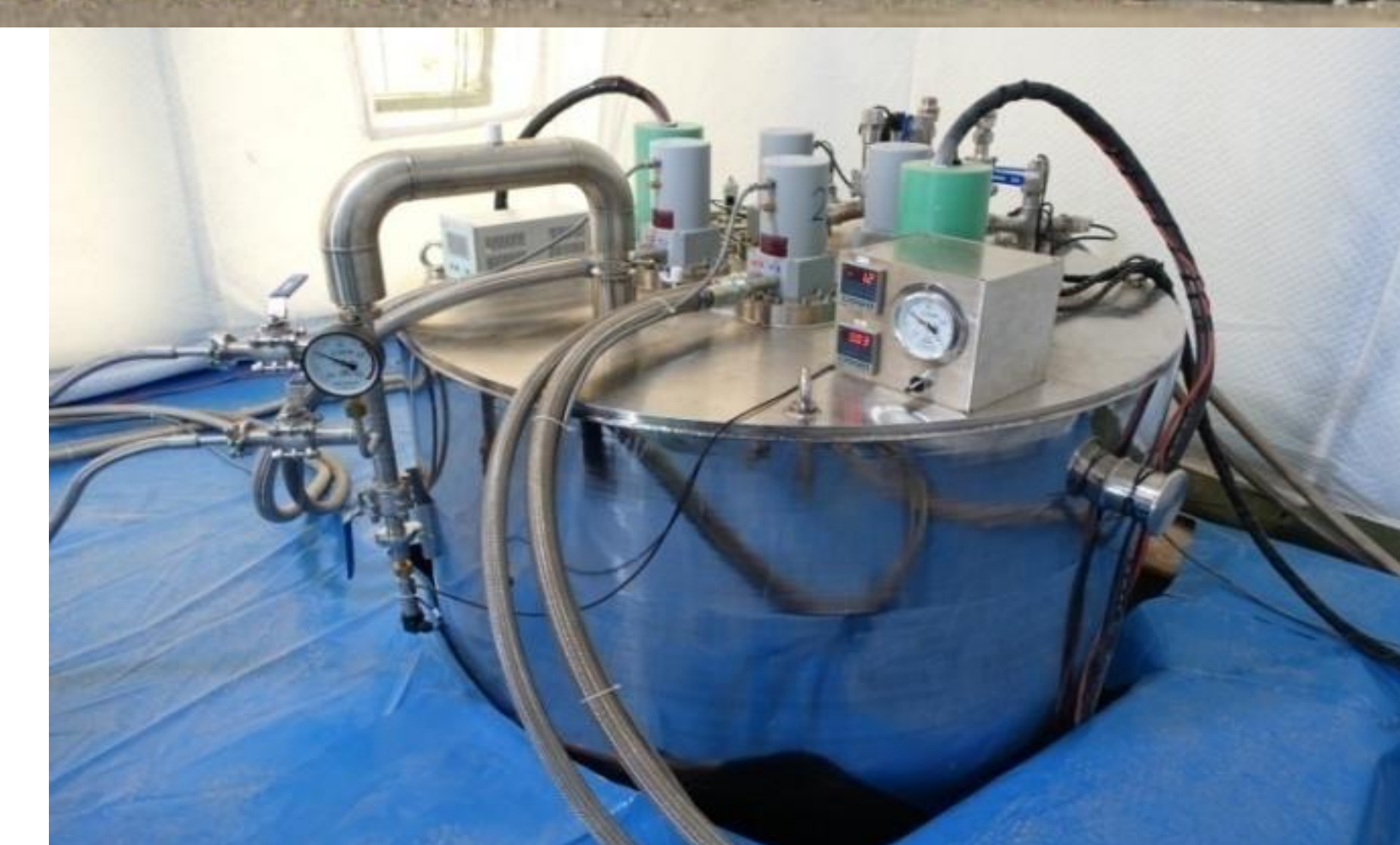
Fig.7. A photo of 1 MJ/1 MVA SMES-FCL installed and put into operation since January 6 of 2017 at a 10.5 kV wind farm locating in Yumen, Gansu Province of China.
