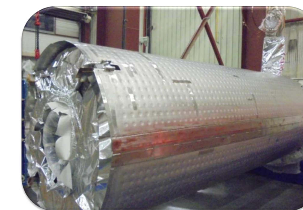
Thermal shield installation (ASME welds & controls, pressure & leak tests)
