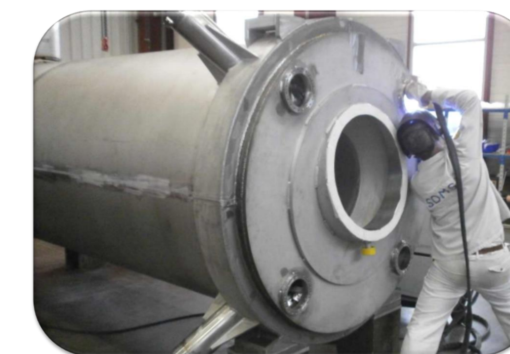
Outer vessel installation (final leak tests on the 3 vessels)
