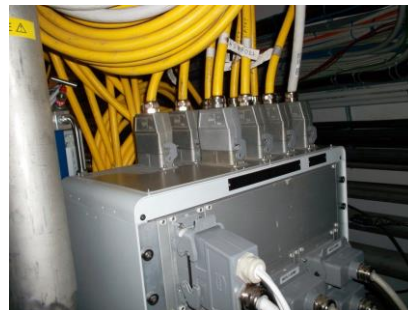
Fig 2. Lemo/Redel S series 51 pin assembly (3.2kV).
