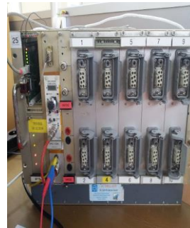
3 kV crate with the new DAQ prototype
