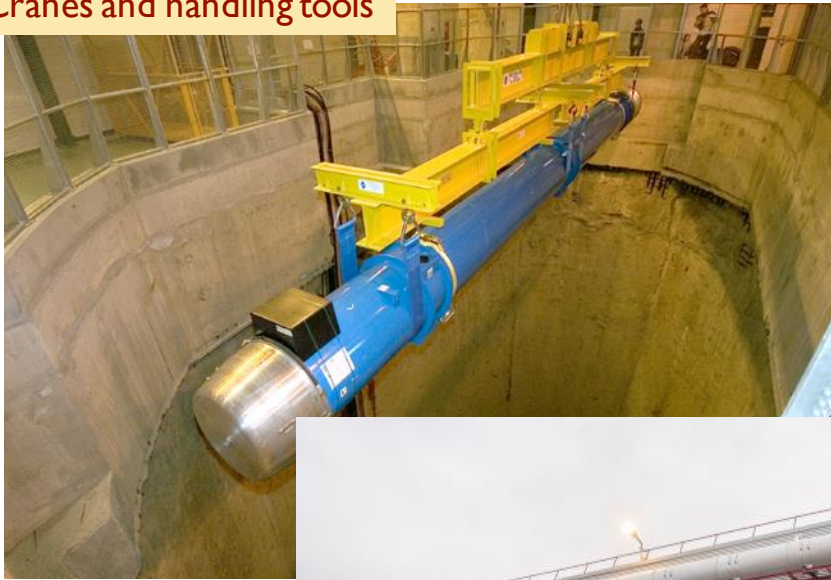
Cranes and handling tools
