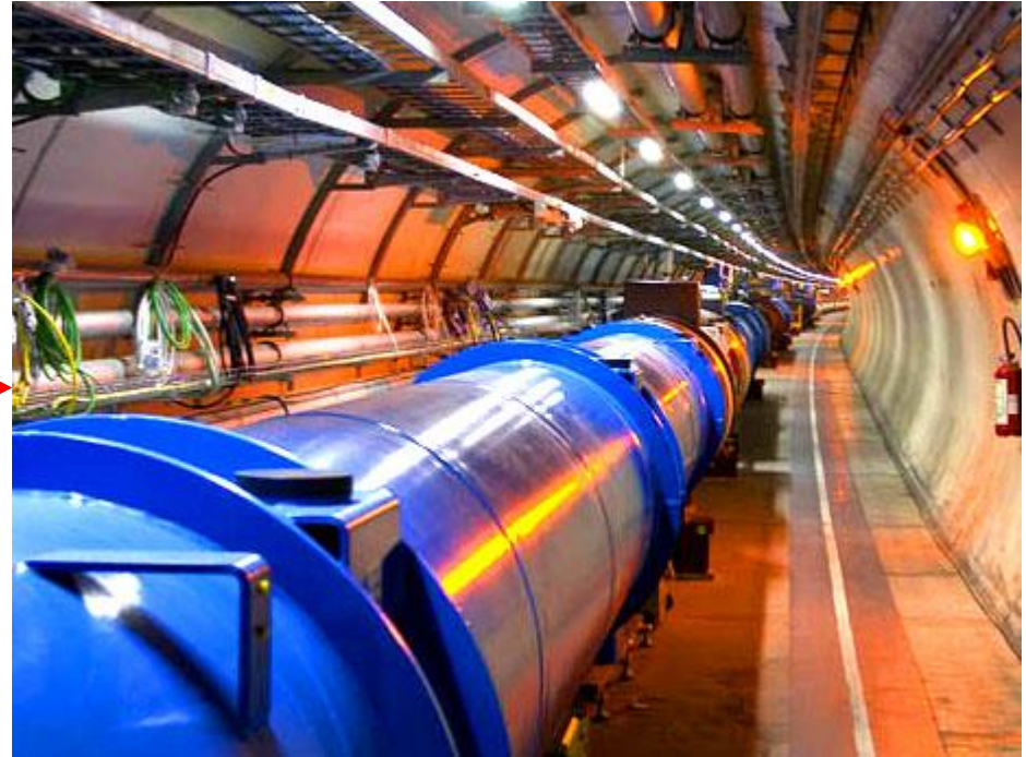
The latest synchrotron (2010) D~9km, E~7TeV
