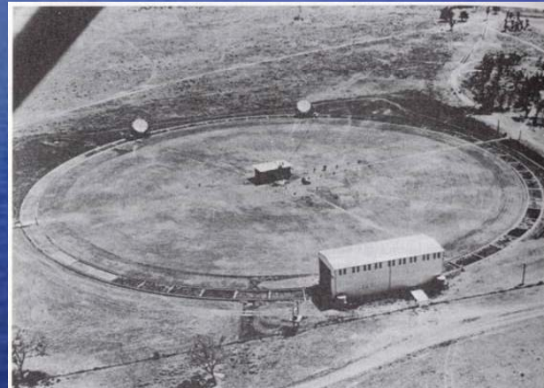
Figure 11.1 Narrabri Observatory in 1963, showing the circular railway track (618 foot diameter), the two optical reflectors (22 foot diameter), the central mast and control room, and the very large garage for the reflectors.
