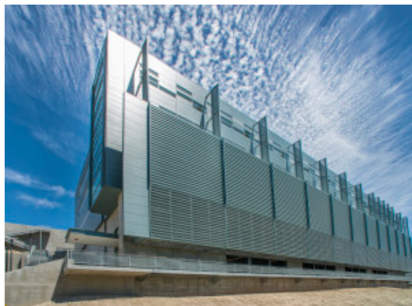
New NERSC machine room at LBNL
