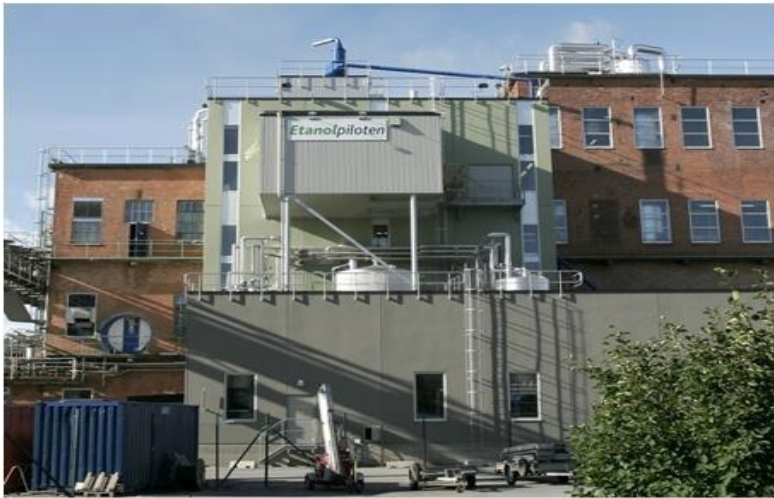
Thermochemical pretreatment of sugarcane bagasse and Norwegian spruce was performed in the Örnsköldsvik demo plant in Sweden (< www.sekab.com >).
