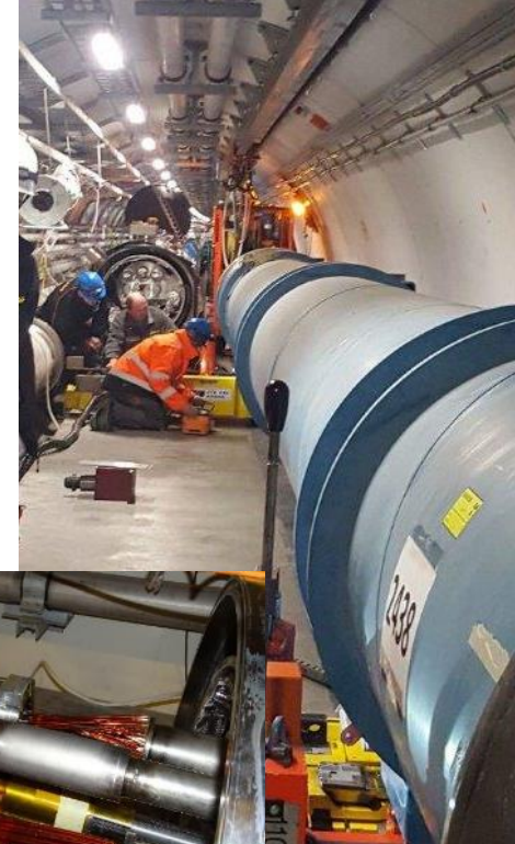
New A31L2 magnet installation
