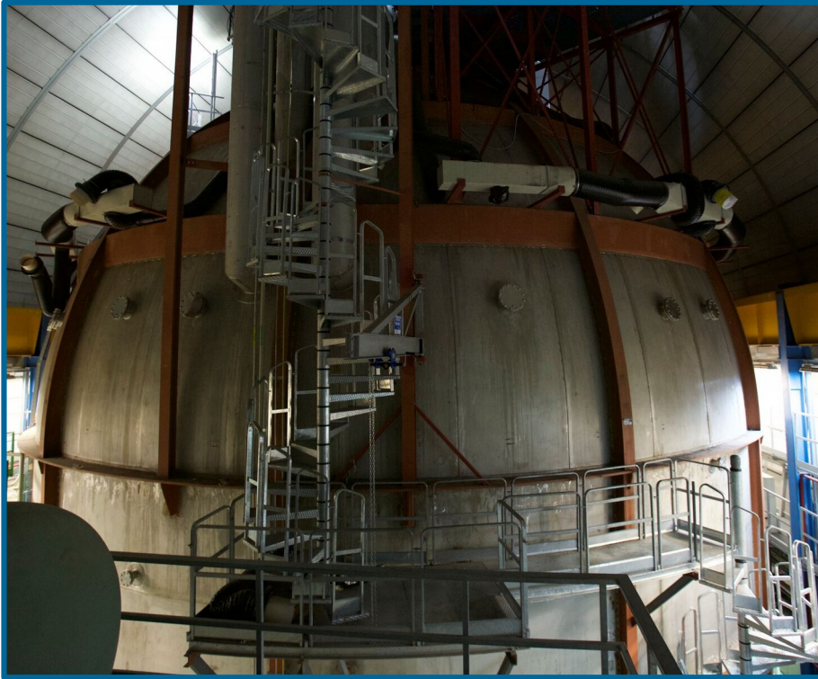
Before thermal insulation
