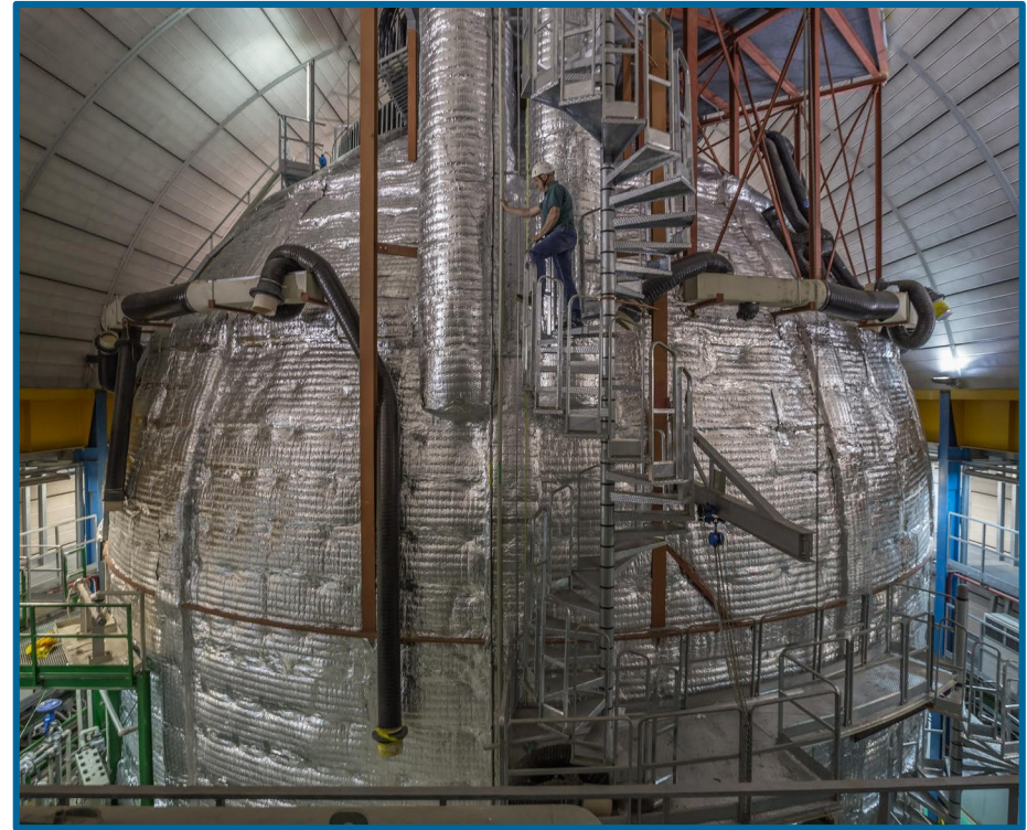
After thermal insulation
