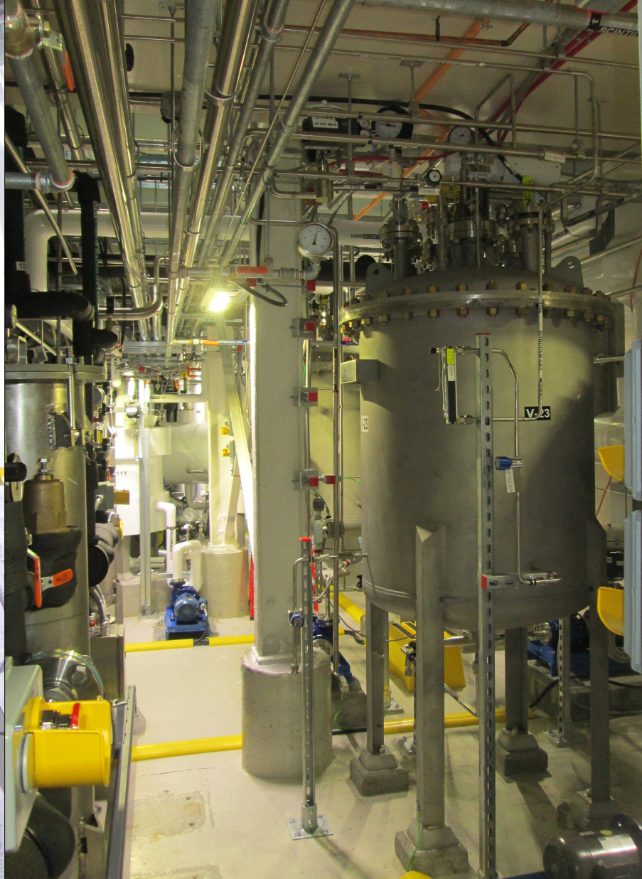
LAB purification plant commissioning underway for scintillator fill late 2017
