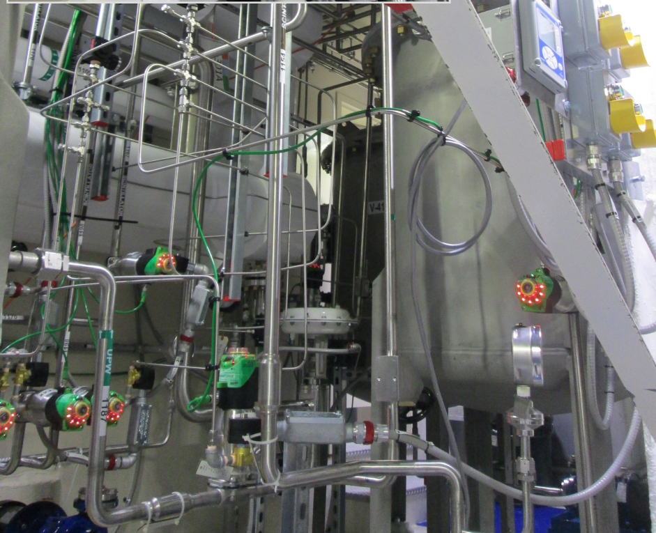
LAB purification plant commissioning underway for scintillator fill late 2017
