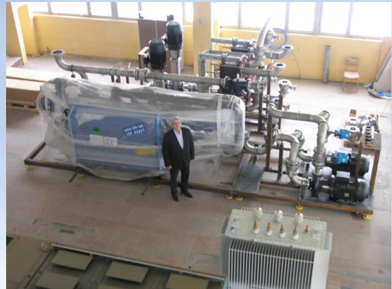
Water cooling system
