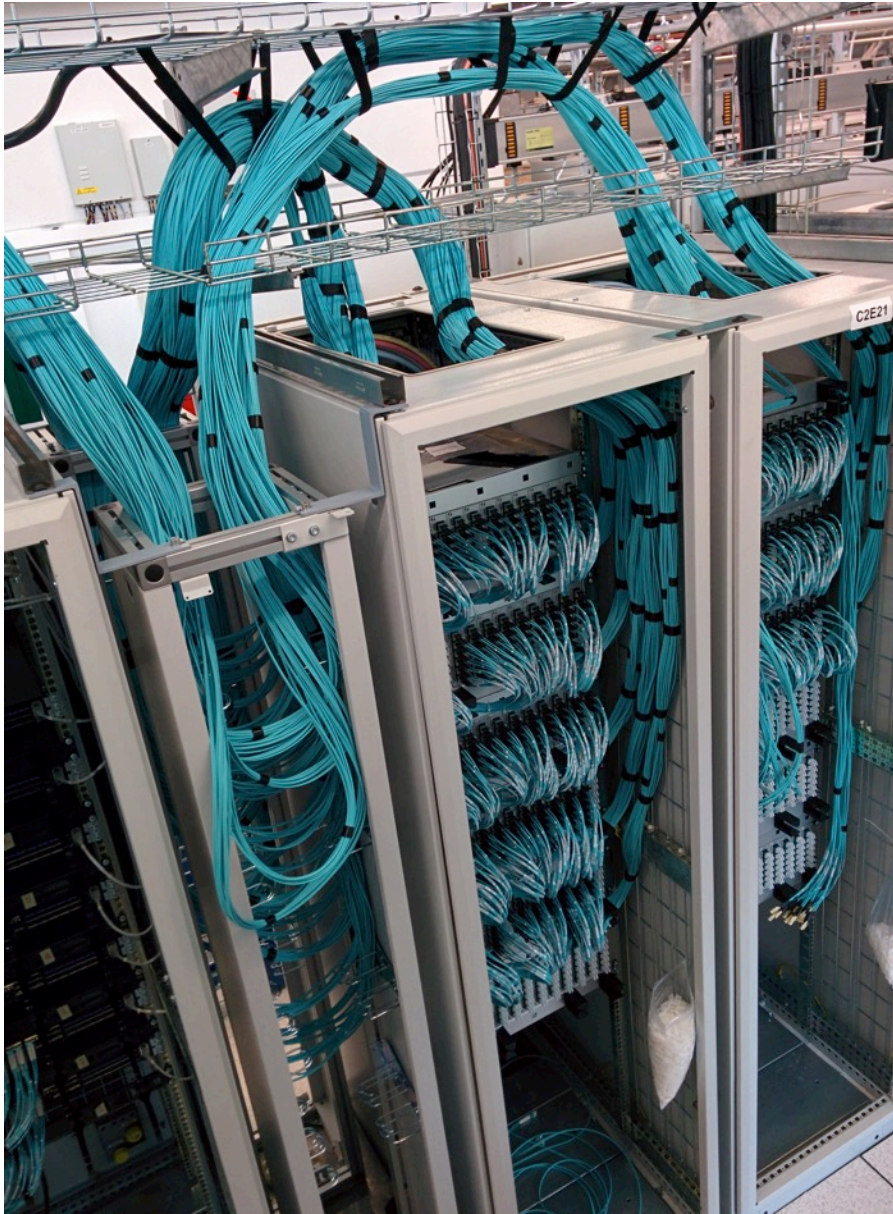
Data concentrator patch panels
