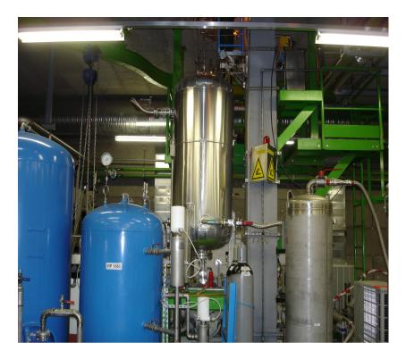
The activated fluorocarbon accumulates in the tank in USA 15. The decay radiation penetrates the tank walls and delivers a certain dose to a person in the vicinity
