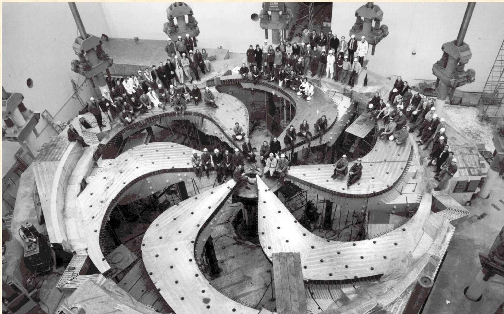
Lower half of the Main Magnet poles
