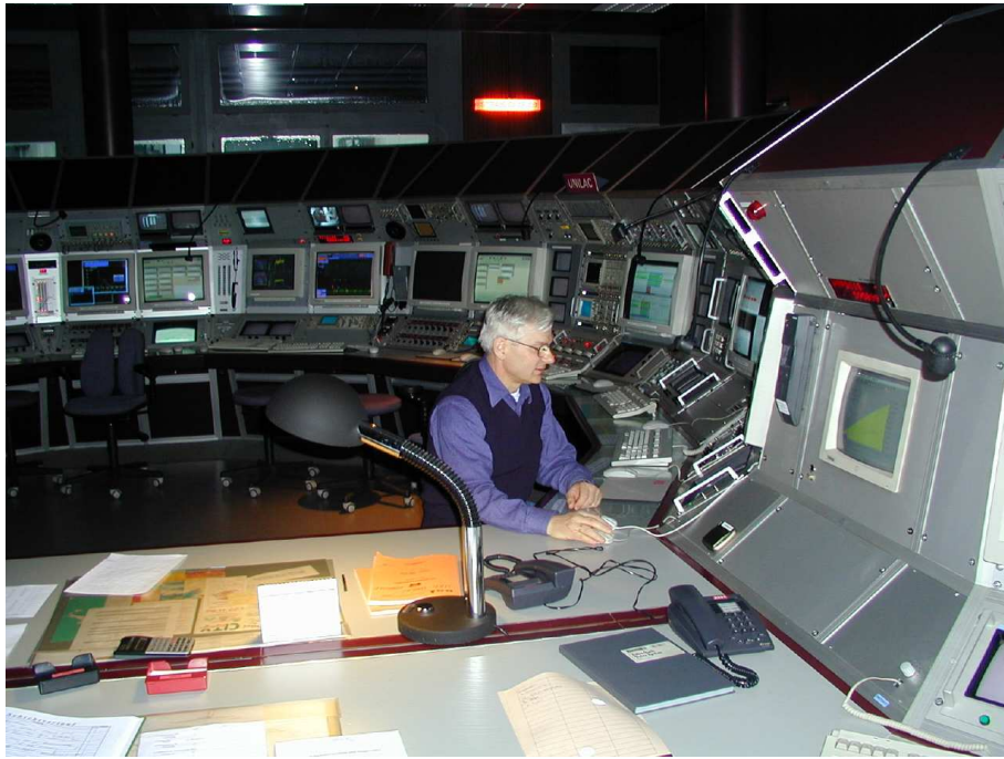
Figure 1.3: One section of the operator control room at GSI.
