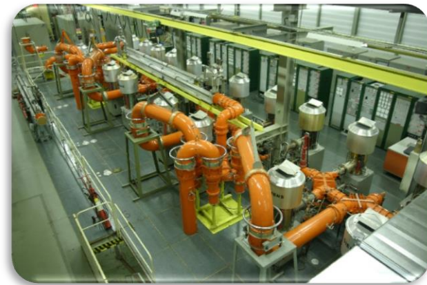
CERN SPS 4 x 500 kW unit One transmitter density = 1.1 kW/m 3
