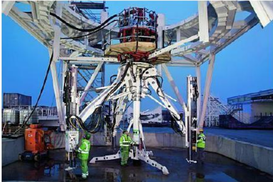
Figure 31: Shaft sinking drill rigs, Nant de Drance (CH)
