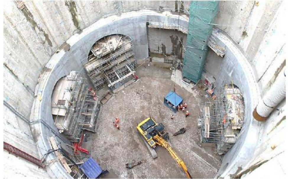
Figure 28: London crossrail shaft, diameter 30 m, depth 45 m
