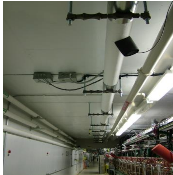
Reference Line in Tunnel
